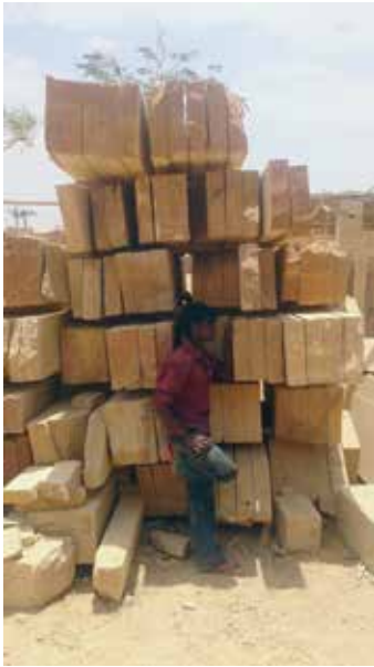
This page, top and top right: the stones were sourced from different quarries, based on the criteria for compressive strength, finish, colour etc for different applications. These massive stone slabs are traditionally stacked on stone pegs similar to our temple construction details. Right and far right: the temple taking shape during its construction phase. Below: the circular opening that forms a halo around the shivlinga idol
