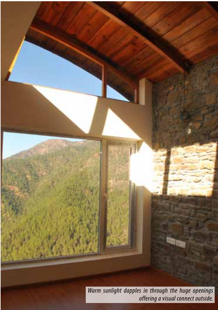
The roof is conceived as a traditional wooden and galvanised iron covering.
