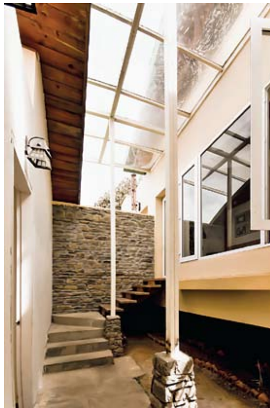
The enclosed courtyard with its glass ceiling not only allows sunshine and daylight but acts as a heat trap as well.
